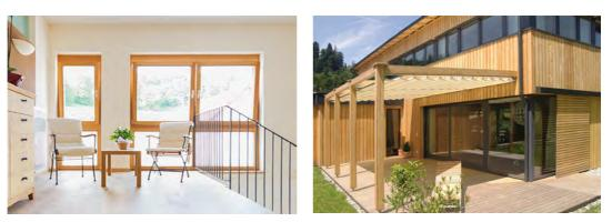
Paarhammer ECO Facade (curtain wall) is constructed with the strength, warmth and energy efficiency of timber inside and aluminium clad for zero maintenance outside. The visible aluminium powder coated profile is clipped onto the outside, is only 50mm wide, available in a variety of colours, and guarantees a hardwearing and maintenance free outer skin.
