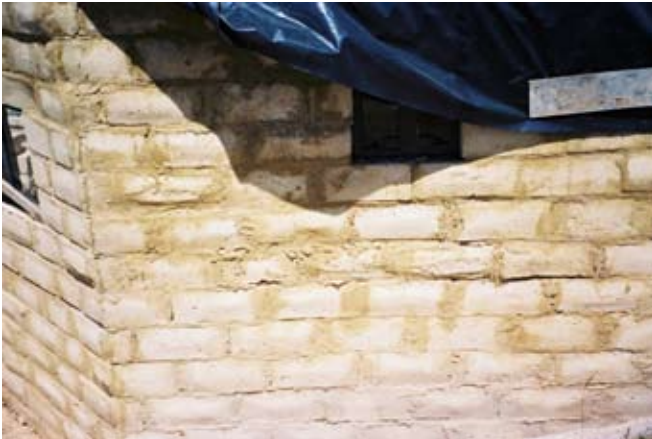
Incorrect laying of Timbercrete Bricks
