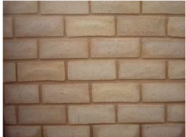
Correct laying of Timbercrete Bricks
