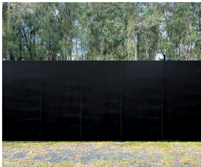
12mm – Temporary hoarding panelling
