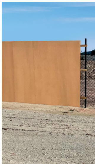
12mm – Temporary hoarding panelling
