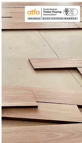
12mm – Timber flooring underlay
